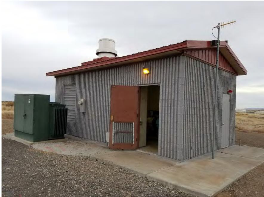
*Facility Conditions:* The metal roof and masonry are in good condition. The wood part of the building is removable and is deteriorating due to weather and time.
