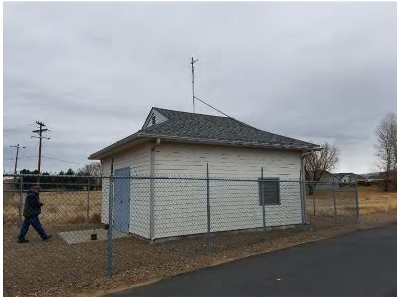
The building has siding and shingle roof. The building is in fair condition inside and out. The louvers allow dust to enter the building causing maintenance problems.
