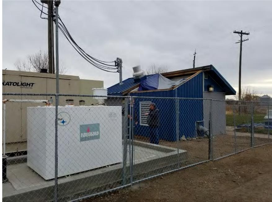
generator is located in a fenced area nearby. An additional secondary containment curb has been added to the aboveground fuel tank since the double wall fuel tank was installed years ago. The pump and motor assembly was under repair at the time of the evaluation. The motor was scheduled to be reinstalled soon. The roof section over the pump was removed and covered with a tarp. The roof is removal for pump maintenance. The roof will be replaced after the pump repair is complete.
