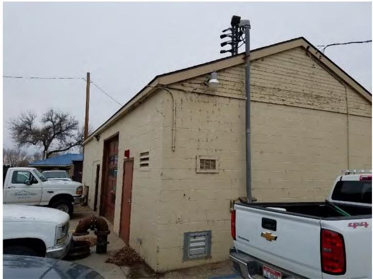
*Facility Conditions:* The building is very old but with ongoing maintenance it is a usable condition. The building does not have air conditioning, but City staff report that the pump runs during the summer without overheating. The electrical system is functional but the condition of conductors and connections is unknown until a thermal image test is complete.
