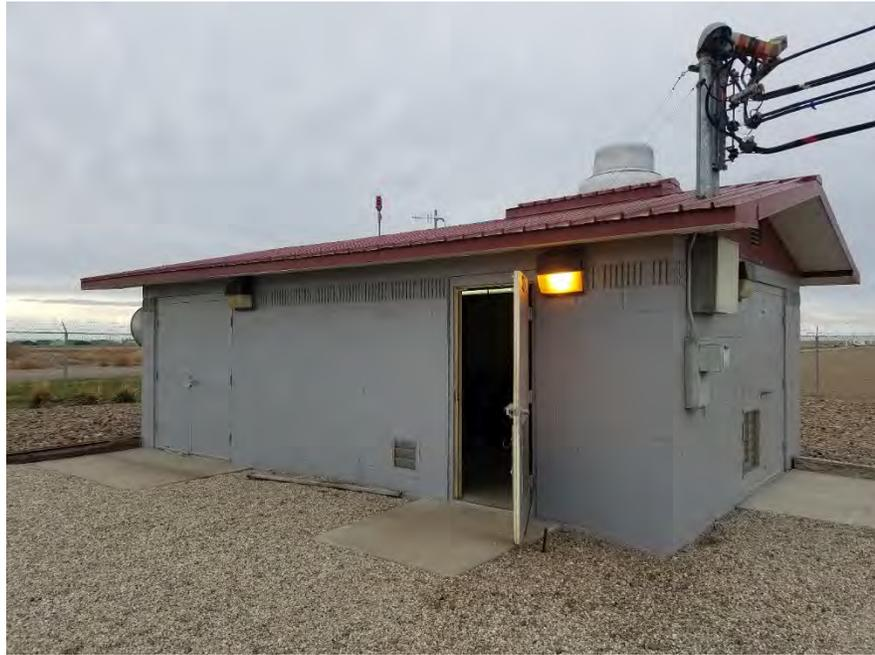
site is fenced with a gate at the road. Power is overhead from a power pole near the road. SCADA system and an antenna on pole next to the roof provide remote monitoring.
